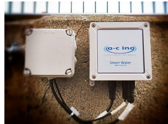
iWesla Flow Meter Mote at Rivas Facilities. Source: iWesla
