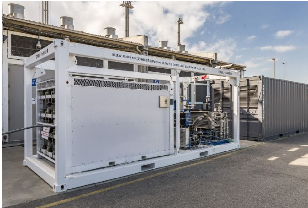
Boeing's reversible solid oxide fuel cell system in operation in Huntington Beach, CA. Photo credit: Boeing.
