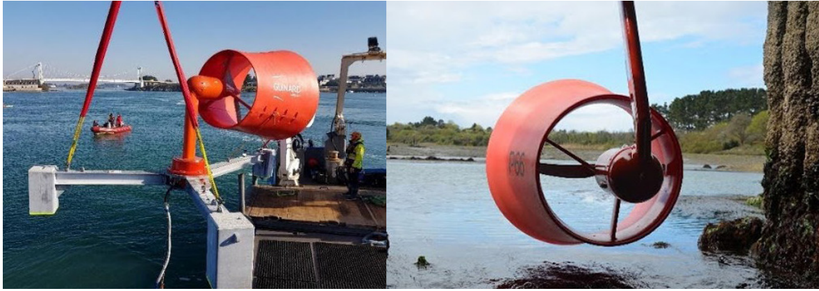
FIGURE 17 Installation of an axial flow HT from Guinard Energies ( photo courtesy of Flavien Martine ). The turbine, installed in a duct, can generate 20 kW.
