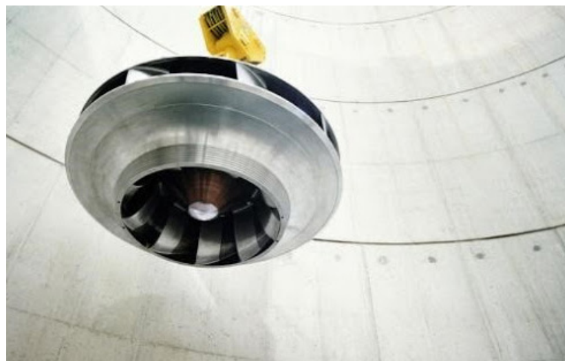
■■■ FIGURE 14 Installation of a pump-turbine. Photo courtesy of Voith GmbH & Co. KGaA.
