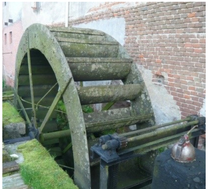
■ ■ ■ FIGURE 4 The existing breastshot water wheels, for which a 1 : 2 scale model was investigated. The original diameter is 4 m.
