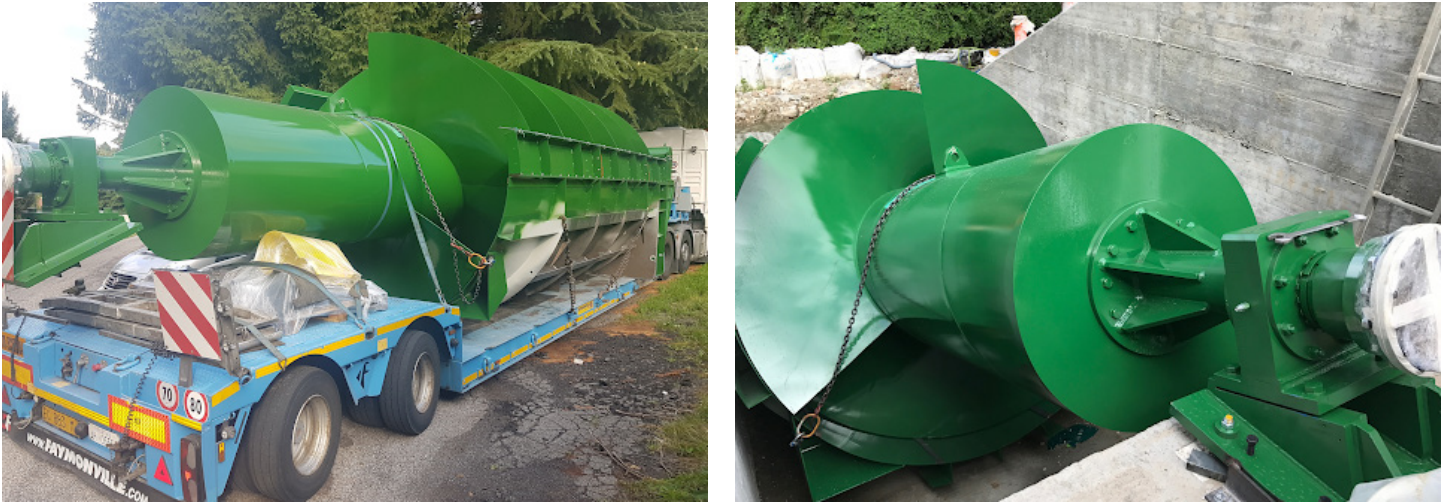
■ ■ ■ FIGURE 9 Hydrodynamic screw installation in Italy (Carmine Fioravante, Artingegneria).
