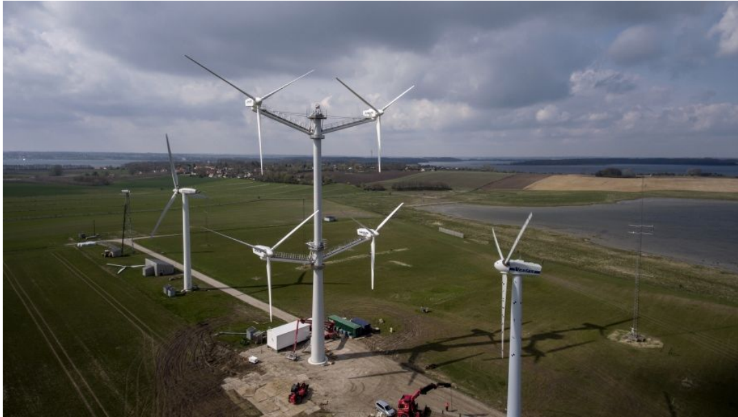
Multi-rotor turbines produce 2% more electricity than conventional turbines. Image Source: Power Technology .
