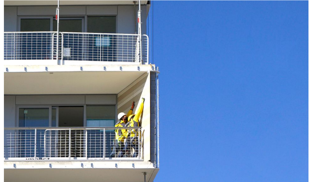
Installation of Mitrex Solar Cladding Building Materials. Image source: Mitrex .
