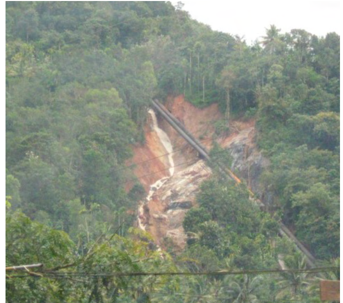
Figure 1(b) Penstock failure at Panniyar Hydroelectric project due to leakage at the joint.
