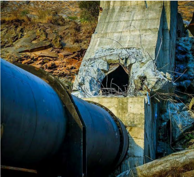
Figure 1(a) Sorang Hydro Power plant accident on November 18, 2015, in Himachal Pradesh, India. It was reported that this failure occurred because of the leakage of penstock, started at an earlier date. In addition, this hydroelectric project is located in a fragile zone where slope destabilization and landslides have been blamed on rainfall fluctuations, floods, and other natural factors.
