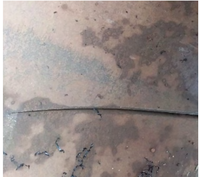
Figure 12(a). Burst pipe at a low pressure region of the pumping main.
