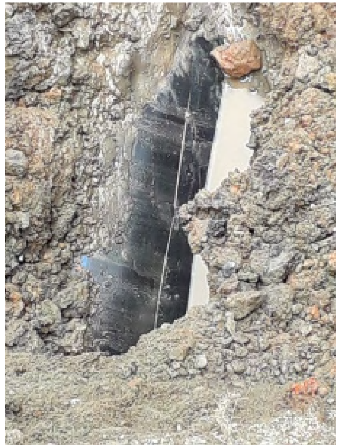
Figure 12(a). Burst pipe at a low pressure region of the pumping main.
