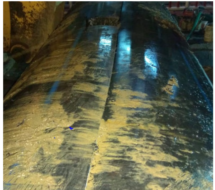
Figure 14. Pipe burst due to malfunctioning of surge protection devices.
